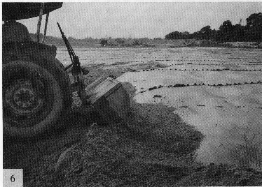
Fig. 6. Sand deposition onto geotextile-bamboo fascine mattress over a slime pond.
