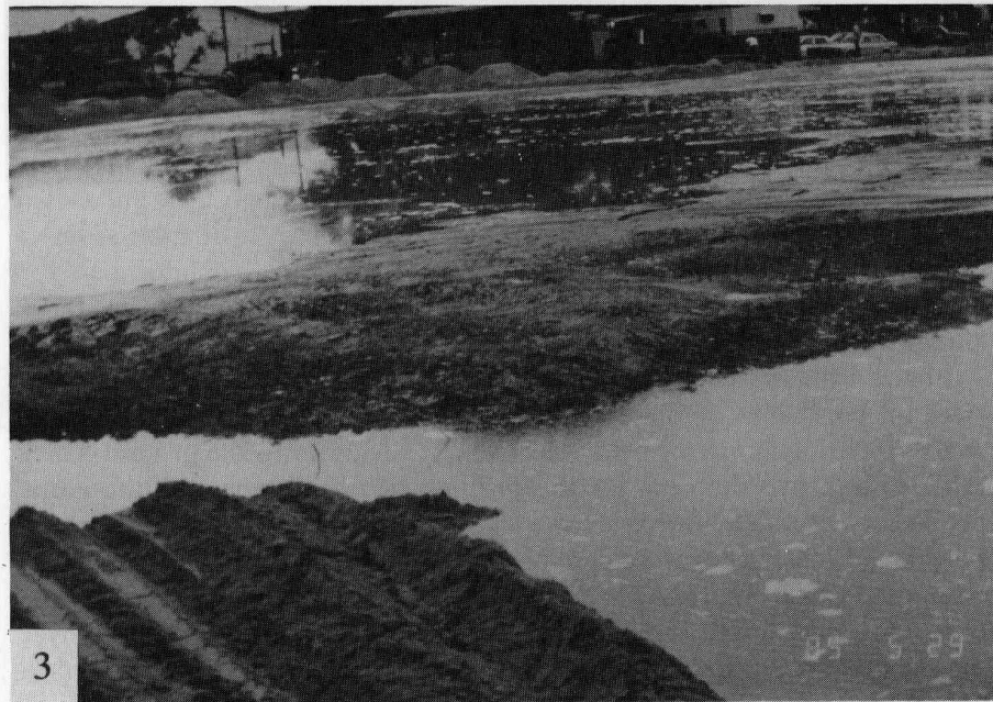
Fig. 3. Mud waves from end tipping into a disused tin-mining slime pond.
