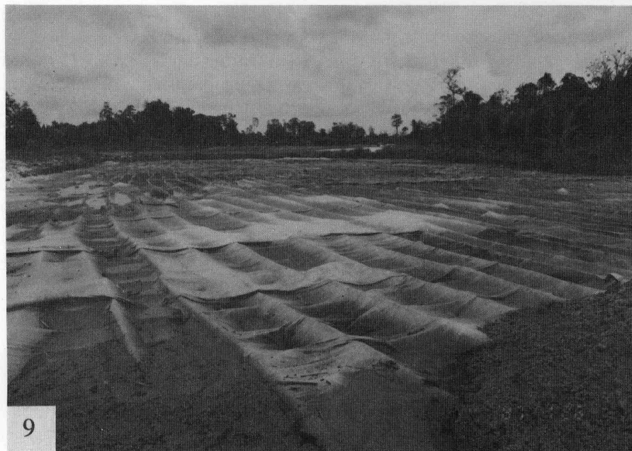
Fig. 9. Geotextile-bamboo fascine mattress over peat.
